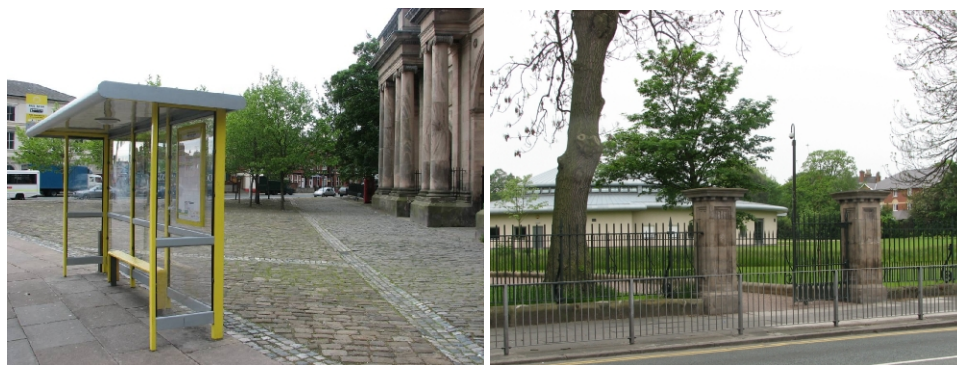
Standard concrete slab paving, bus stop and unpainted galvanised railings, all compromising the setting of the conservation area and detracting from key architectural elements.
