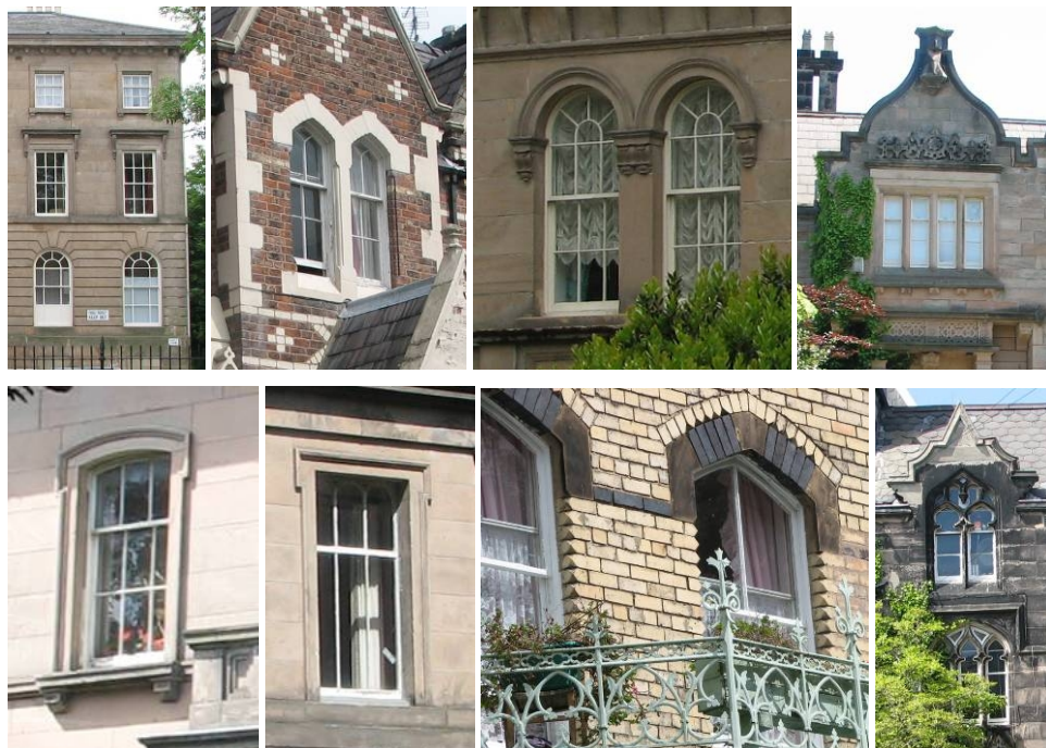
Windows within Birkenhead Park Conservation Area
