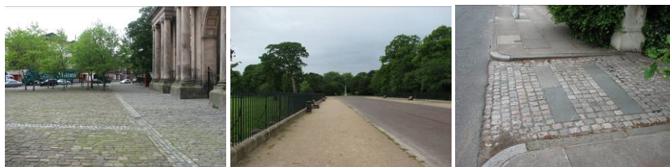
(Left) setts to the front of the Grand Entrance; (middle) compacted gravel to the footpaths within the park; (right) setts and stone slabs to a driveway entrance
