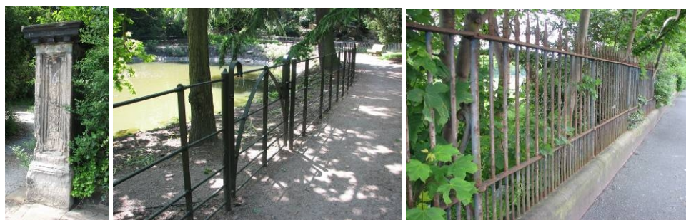
(Left) Original gatepost; (middle) new estate railings and gate around the Lower Park lake; (right) original railings and repaired plinth wall.
