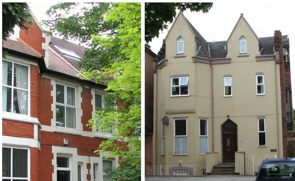
(Left) photograph showing the detrimental effect replacing roof coverings can have on the appearance of a pair of buildings and the awkward detail it results in at the join; (right) a late 19 th century building that is barely recognisable as such as a result of changes including the installation of UPVC casement windows, the rendering of the front façade and the use as concrete pantiles as a roof covering.
